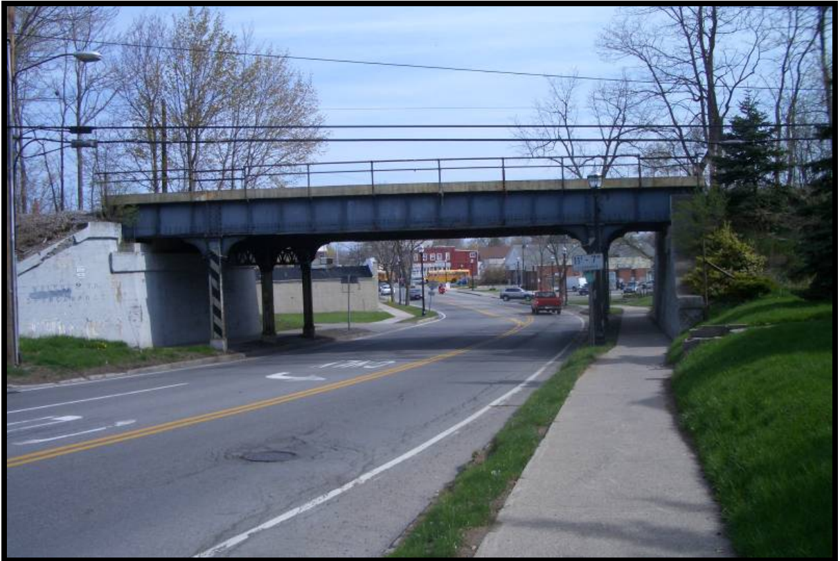
Photo 4: View of the CSX railroad bridge facing north. The bridge crosses South Union Street.
