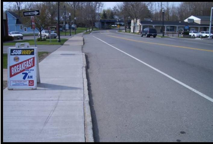
Photo 9: Shoulders on South Union Street facing south. Note the condition of the roadway, curbs, and sidewalks.
