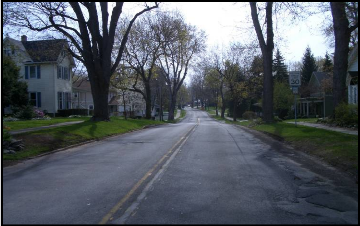
Photo 6: View eastward along Lyell Avenue. Note condition of the road, the curbs, and location of the sidewalks.
