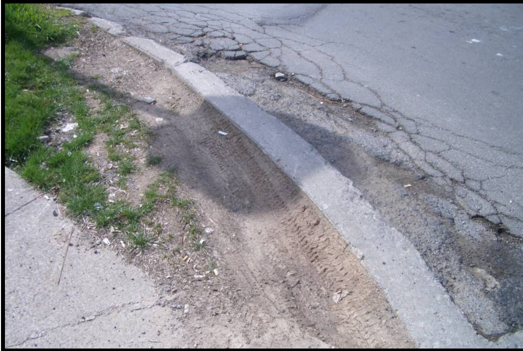
Photo 8: Curb at the intersection of Lyell Avenue and South Union Street. Note the condition of the pavement and curb, as well as the tire marks indicating this curb is breached regularly.
