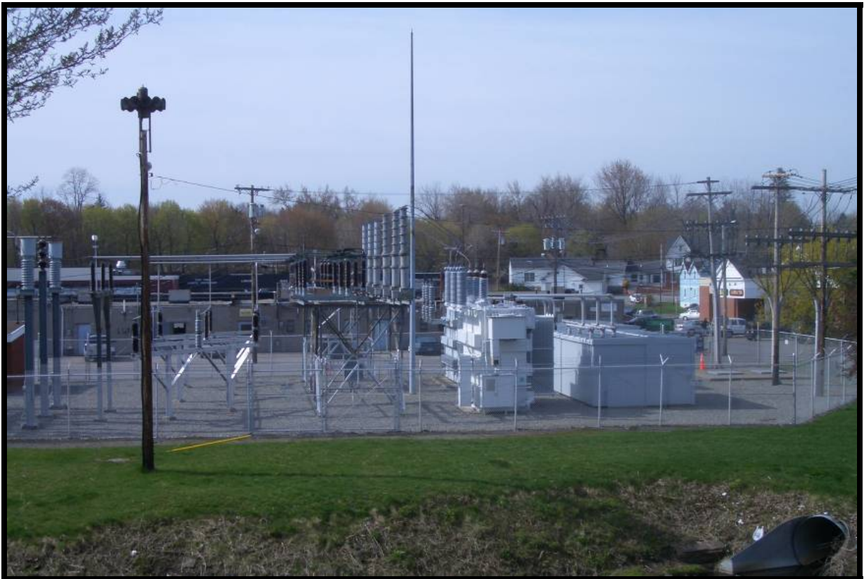
Photo 16: The Village’s electric facility located in the Village Plaza between Northrup Creek and East Avenue.
